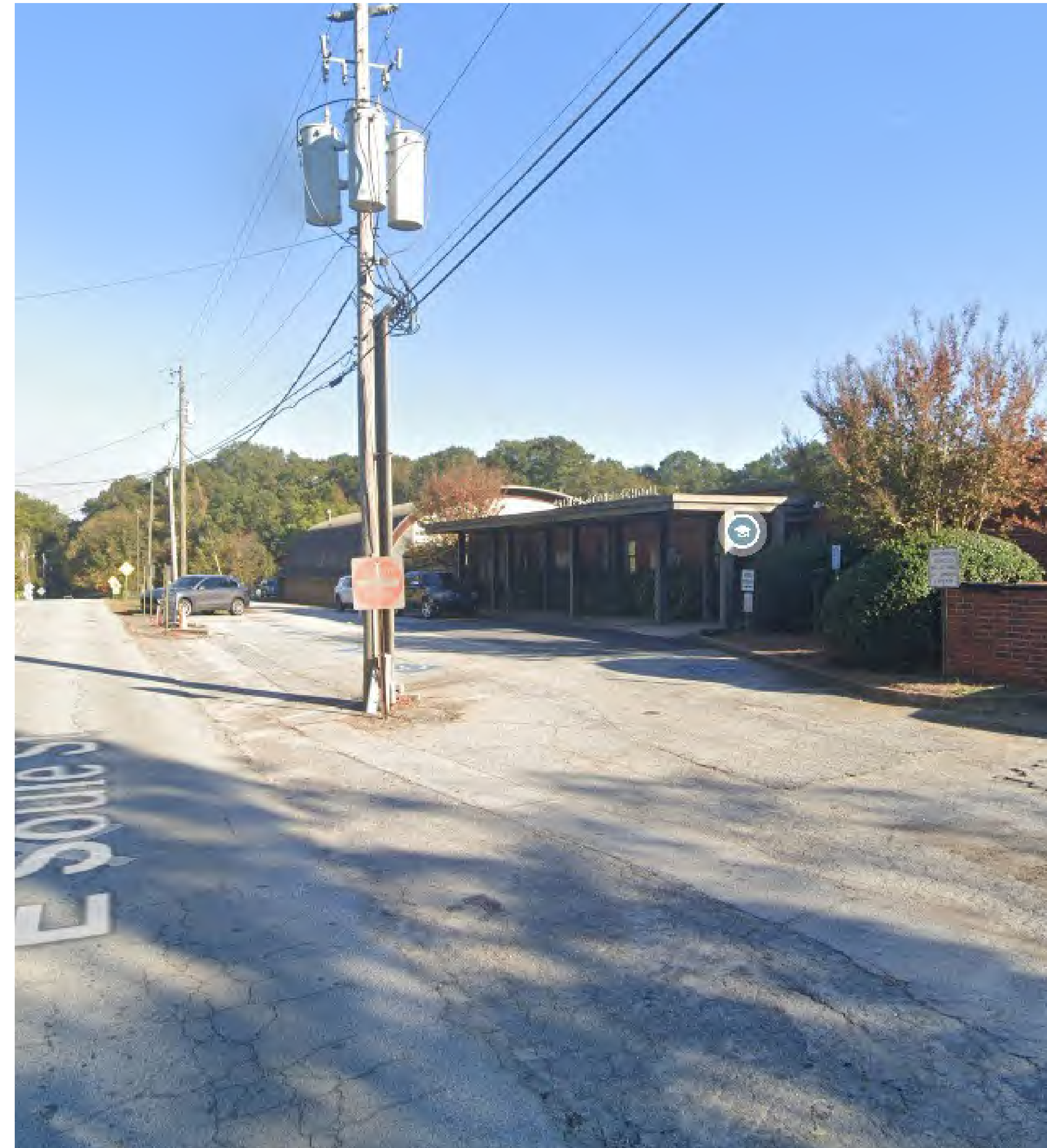
FRONT OF PALMER STONE ELEMENTARY SCHOOL
